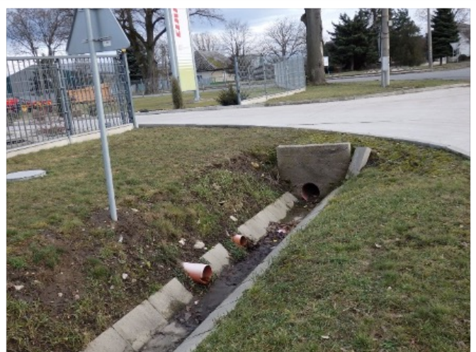
Draining rainwater in the township of Zemplínsky Klečenov (Trebišov). Concrete stream channel. Culvert. Unsustainable channelization and inadequate stream crossings alter hydrology and destroy aquatic life.
