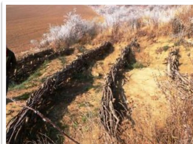
Cascade of small barrier dams. Sustainable solutions, using local by-product branches.
