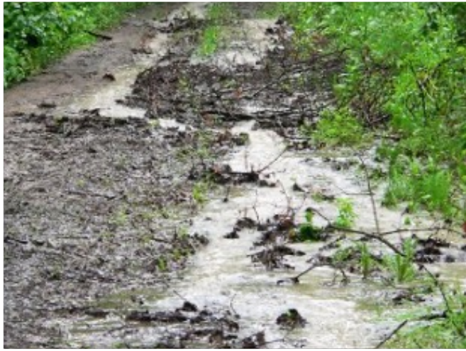
After the flood, waters carried the sediment away, depositing it downstream, eroding the road.
