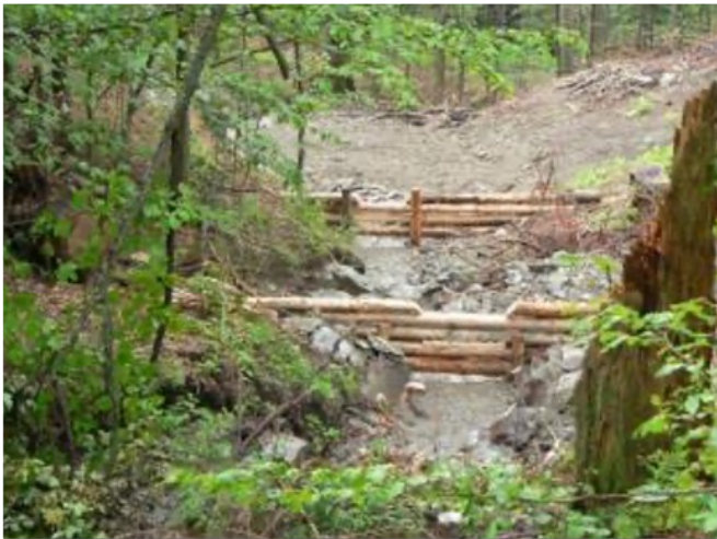
Log dams cascade repairing an erosion gully.
