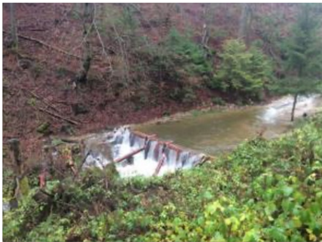
Log dam slows down the kinetic energy of the stream, preventing erosion. The height of the log dam allows fish to migrate. The picture on the right shows the same location upstream.
