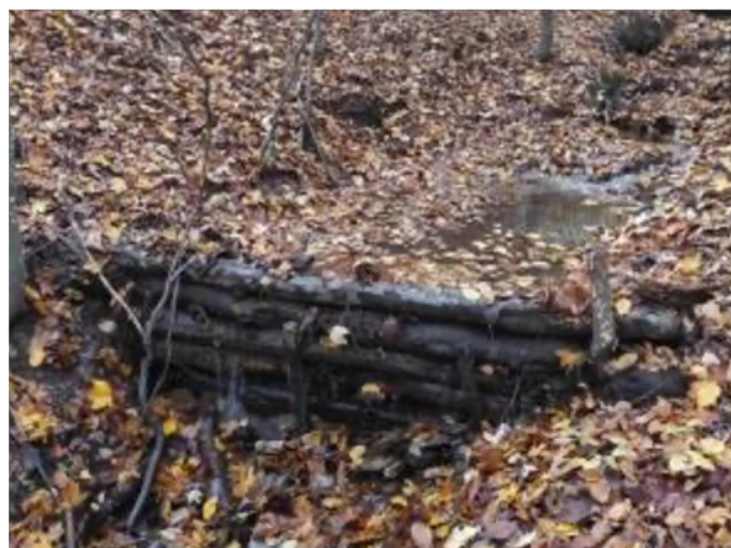
Volunteers construct a log dam to restore the erosion ravine.
